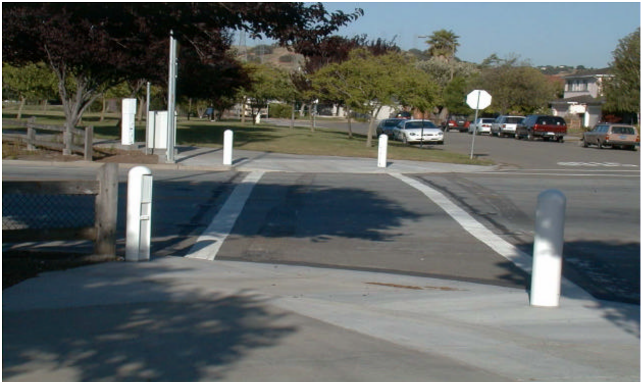
Figure 4: Bollard activation system
