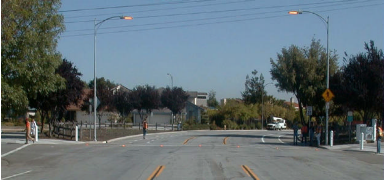
Figure 3: McAbee Road and Golden Oak Way embedded pavement flashing light system
