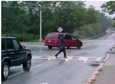
Crosswalk with in-pavement LED system
