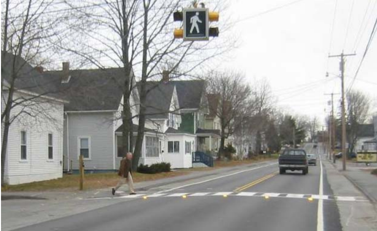
Figure 3 Center Street, Old Town—which also has a time-actuated, overhead school-crossing light
