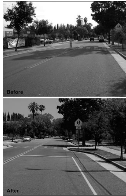
Figure 5. Before and after photos at the mid-block crossing in front of a school showing new curb extensions and updated signage.
