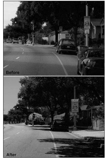
Figure 6. Before and after photos of updated signage, showing use of a larger expressway-sized speed limit plate for the arterial frontage and a FYG SCHOOL plate.
