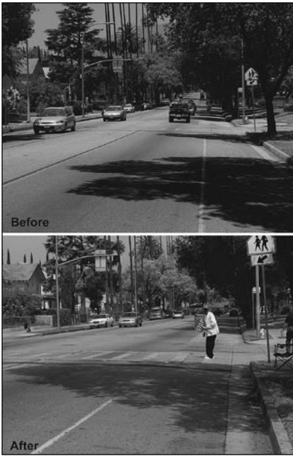
Figure 4. Before and after photos of a lighted crosswalk installed at an intersection near a school.
